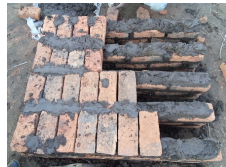
Figure 5) Aerial view of the slits on the base during construction
