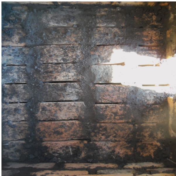
Figure 2) Internal base of the kiln to allow air flow in for carbonation.
