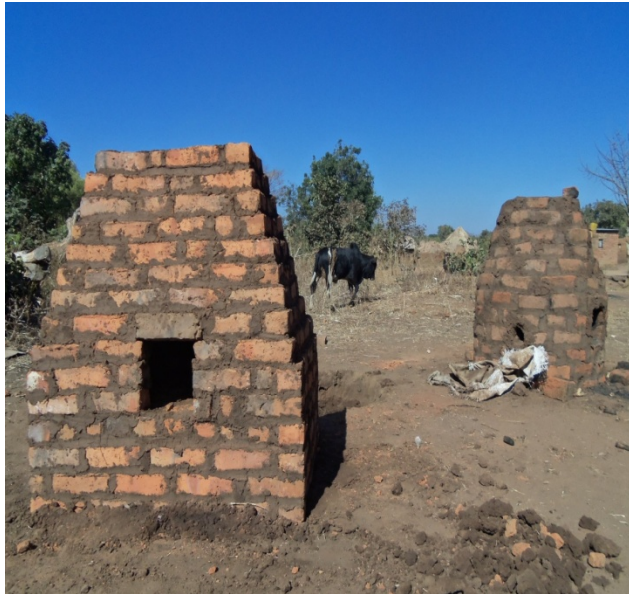
Figure 1) Final kiln (left) designed and constructed by team and community members
