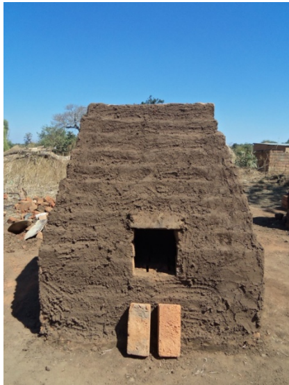
Figure 6) Mud-plastered kiln to prevent air flow through the cracks between the layered bricks during carbonation
