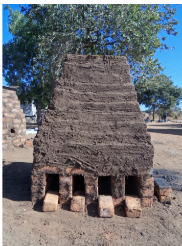
Figure 4) Side view of brick kiln showing air inlets at the base
