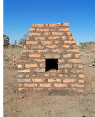
Figure 3) Tapered shape brick kiln
