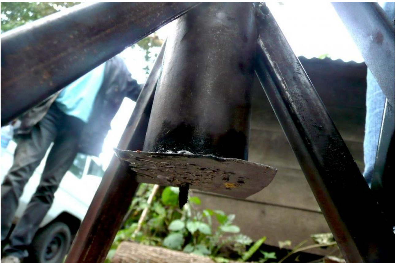
CLOGGED OUTLET HOLES IN THE HAMMER PRESS
